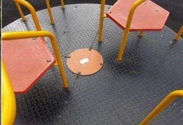
Finding: The bearing is showing signs of wear
