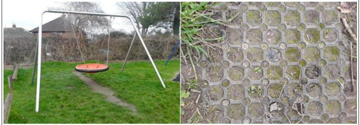
**Finding:** Fixing Pins have been installed in the impact areas **Action:** Remove pins from impact areas of the grass mats
