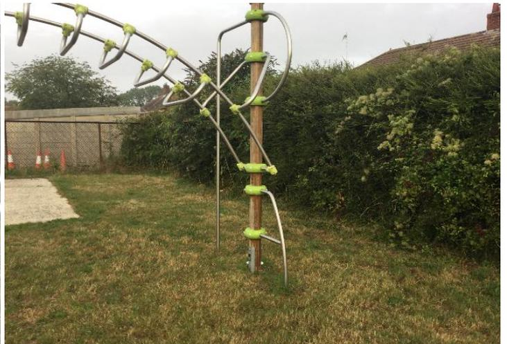
**Finding:** Movement between metal shoe and timber on 2 legs
