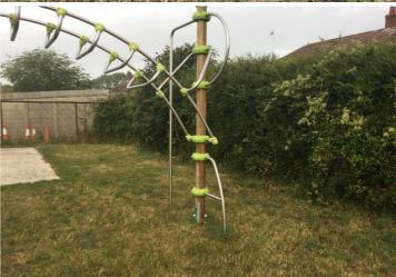
**Finding:** Movement between metal shoe and timber on 2 legs
