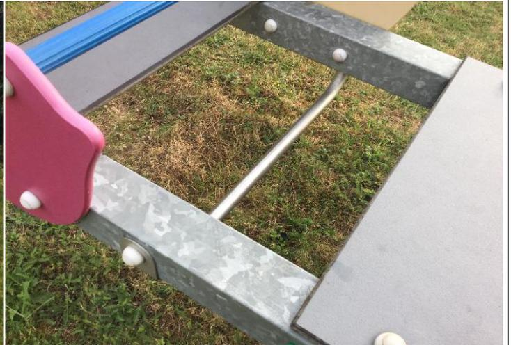
**Finding:** Loose fixings on foot bar
