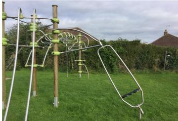
**Finding:** Timber leg has some twist movement which needs **Action:** Investigate timber leg and replace if necessary further investigation
