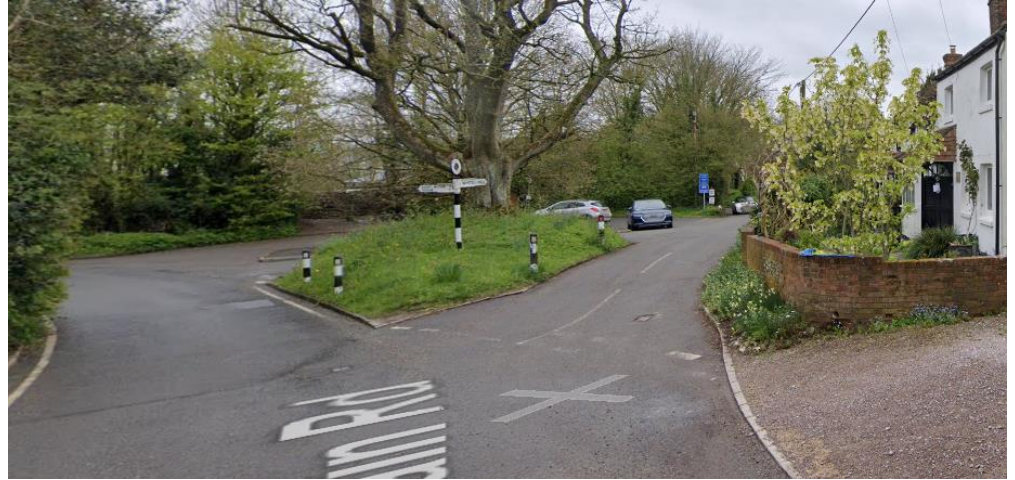
Point 11: traffic island opposite Yew Tree Cottages, looking west.
