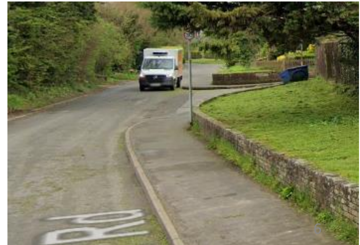
Point 6: Main Road looking West at Hilly Close
