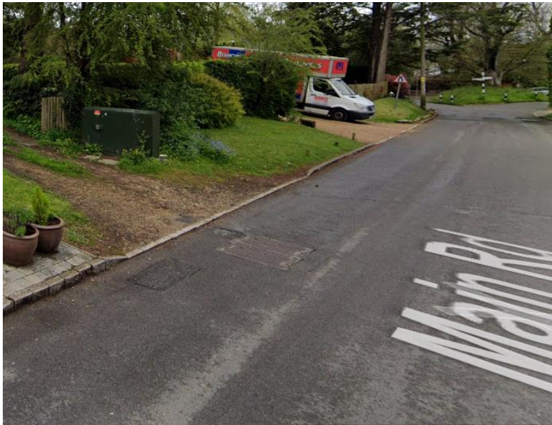
Point 10: BT telecoms hut access track, looking west.
