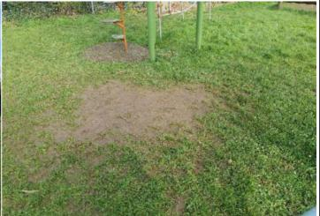
Finding: The grass has eroded within the impact area of the Action: Reinstate the grass or provide an all weather equipment and may not provide the necessary impact surface attenuating properties for the equipment fall height; the surface may also be slippery in wet weather
