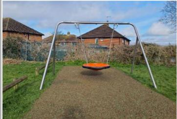
Finding: The seat protection joint cover is missing
