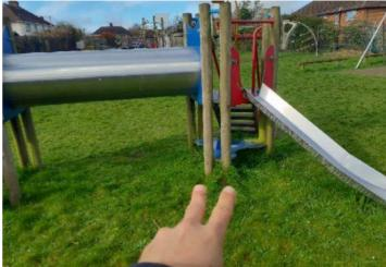
**Finding:** There are 2x timber posts on the structure that have rotted
