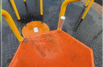
**Finding:** There is/are finger entrapment/s in the seat and the item fails to meet the requirements of BS EN 1176 Part 1 4.2.7.6 Entrapment of fingers
