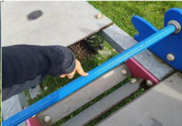
**Finding:** The Handgrips/Footrests rotate and may cause an **Action:** Secure Handgrips/Footrests to prevent rotation. unexpected movement for the user
